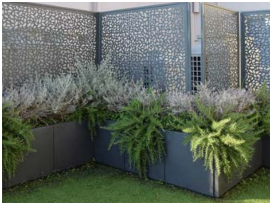
Pannelli frangi vista in metallo zincato e verniciato antracite Overlooking panels in galvanized metal and anthracite painted
